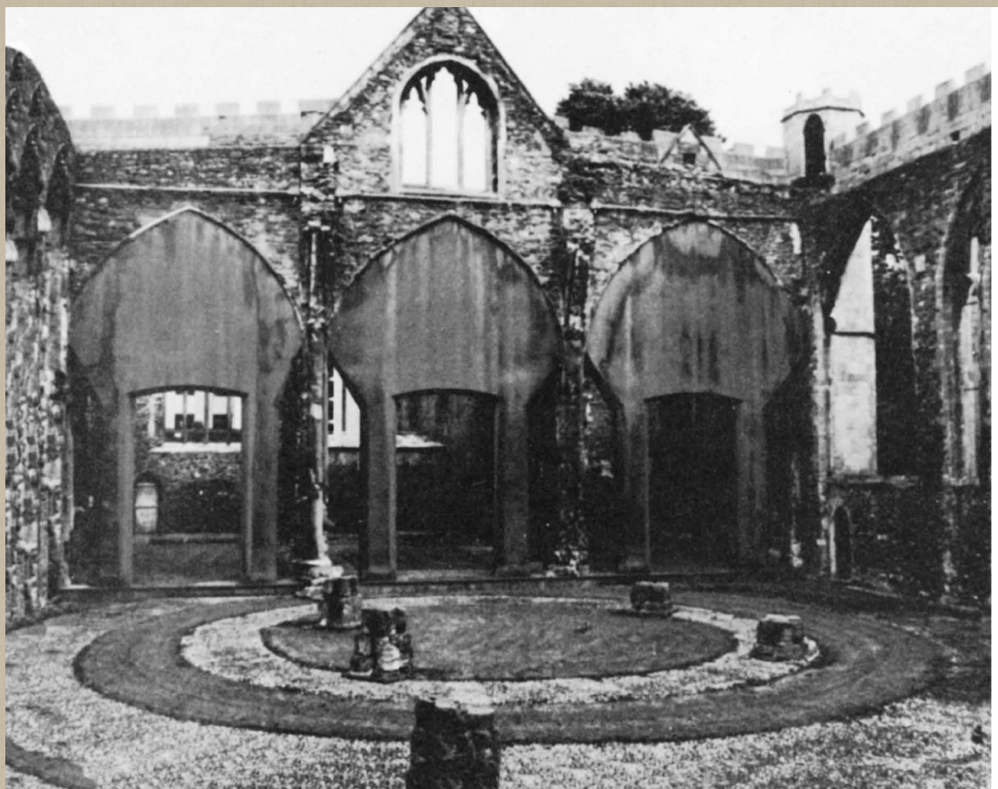
13 Bristol, Temple Church, showing the foundations of a circular church of the Templars which was also demolished by the Order of St John in the fourteenth century and was rebuilt in more conventional style.
