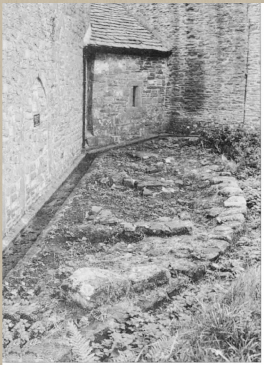
12 Garway, showing the foundations of the original circular Templar church, demolished by the Order of St John, which built a conventional rectangular structure in its place.
